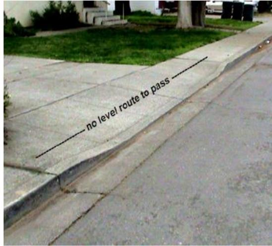
Older driveway ramps cut through the sidewalk at a steep angle. The newer design solves the problem by reducing the angle (and makes driving in more bumpy). New ramps leave a less than 2 degree slope pathway for pedestrians. The older ramps are a difficult problem to solve. The ramps are numerous, and expensive to redesign and replace, in part because they cross onto private property. The result is that people in wheelchairs tend to travel in the street.
